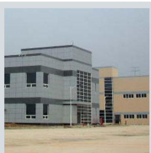
Wuxi Plant (China)
